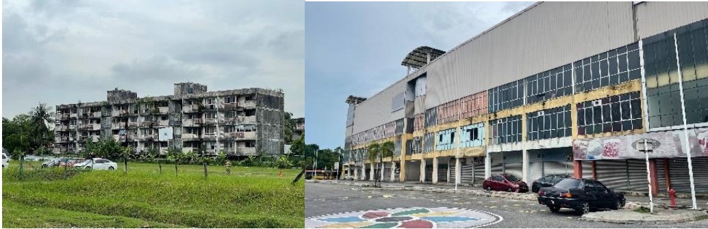
Figure 3. Examples of abandoned and underutilised buildings observed in Southport, Port Klang. Source: Field observation by authors (2026).
